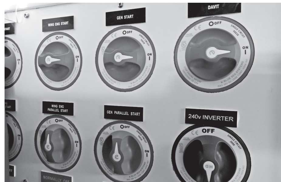
Swapping out Dirona's ship's service selector switch allows the operator to feed the 240V breaker panel from either shorepower or the generator.
