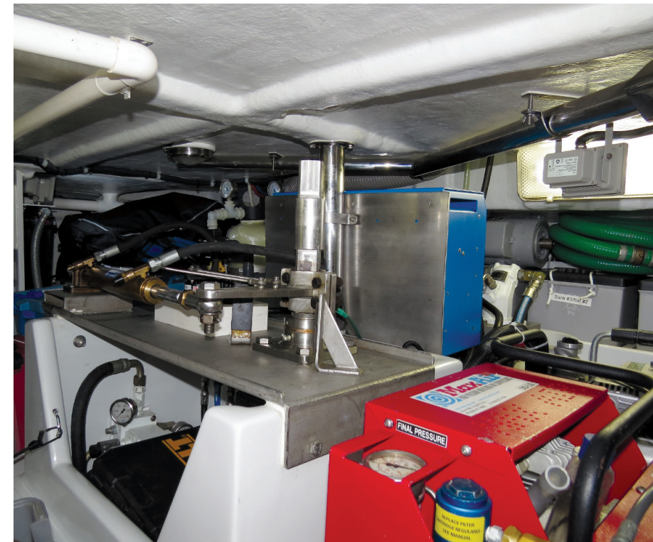
A look below reveals the extensive surgery needed to improve Dirona's genset.
